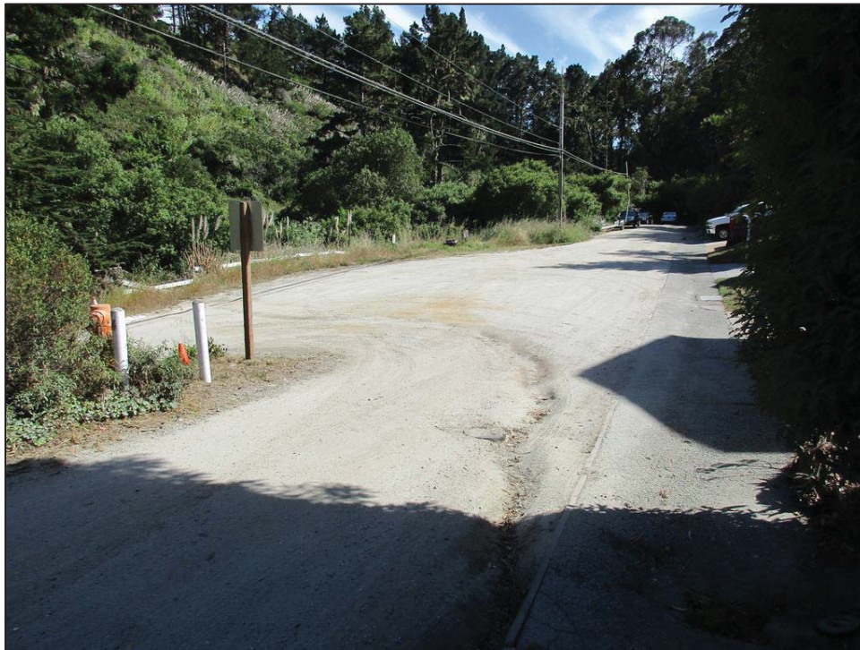
Photo 4: View looking south showing the drainage swale crossing Cedar Street and conveying surface flows eastward toward the unnamed creek.
