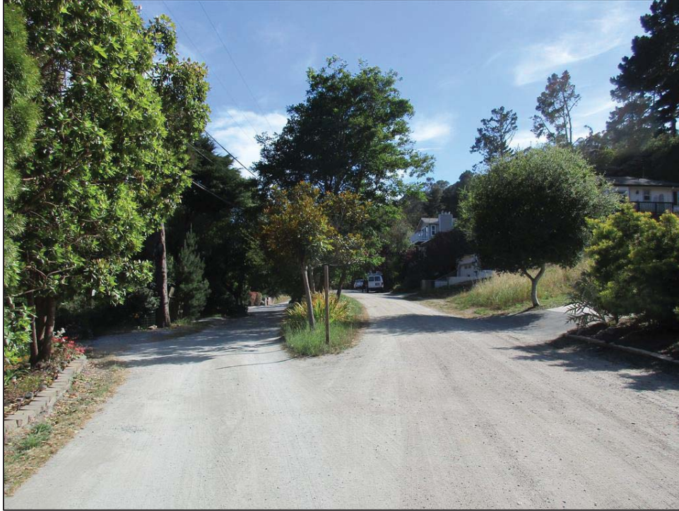
Photo 1: View looking south from the northern side of Cedar Street.
