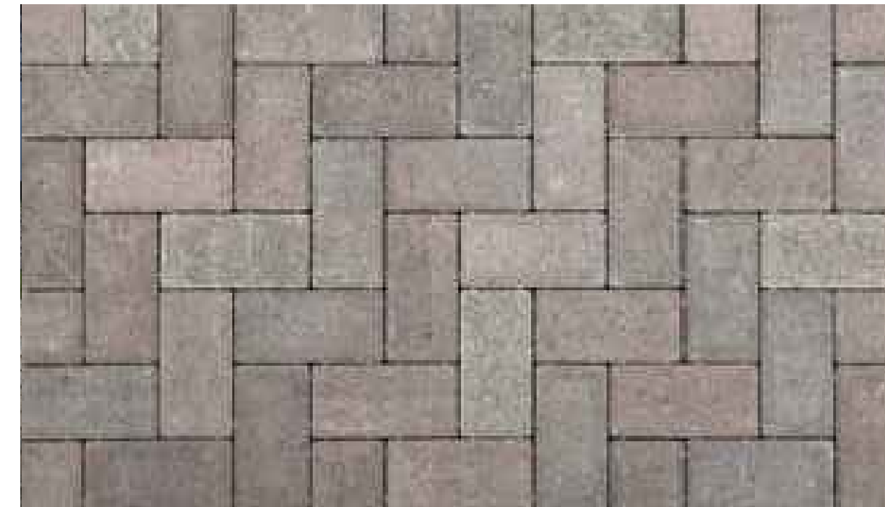
PERMEABLE PAVERS AT DRIVEWAYS (HERRINGBONE PATTERN)
