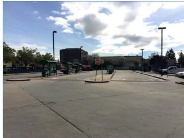
Bus Station Showing Triple Bus Bays
