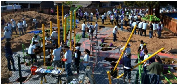
Morning of Build Day, March 21 st
