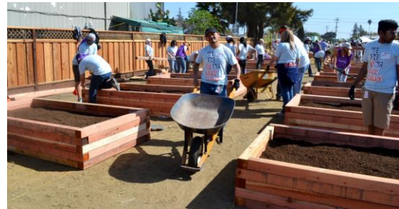
Morning of Build Day, March 21 st
