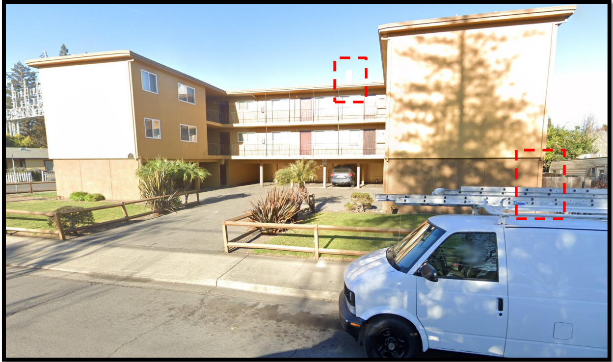
Figure 1 Location of Existing rooftop Antenna and ground cabinets
