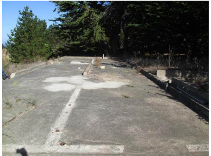
22. View of a concrete building foundation
