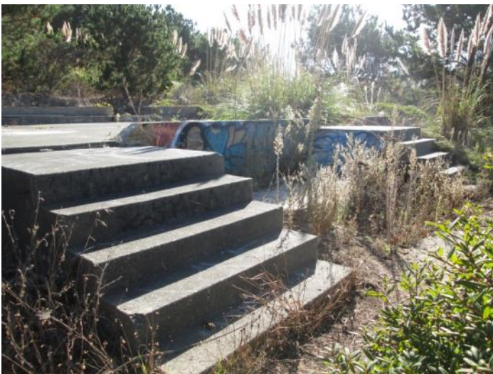
23. View of concrete stairs leading up to a concrete building foundation
