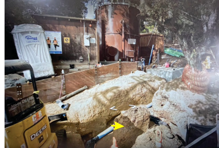
Photo 5. Northwest view of 2020 construction of water tank and booster pump at Cal Water Service Station 112 across from 742 Loma Ct. About 50 feet of new 6" diameter pressure line pipe was connected to the pre-existing line installed some time before 1985. Arrow points to trench exposure of soil similar to that reportedly underlying the landslide on 13 Los Cerros Rd. and 738 Loma Ct.
