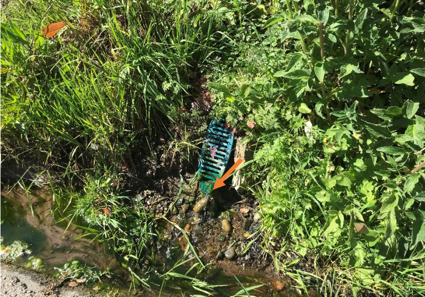
PHOTO 4: Spring pipe at bottom of landslide area: constant spring water flow
