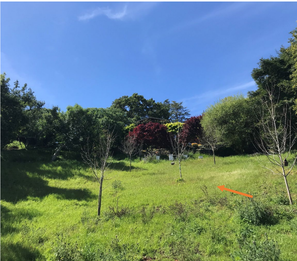
PHOTO 7: Repaired landslide area
