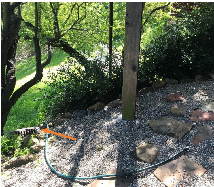
PHOTO 3: Area drain at end of flagstone and gravel walkway
