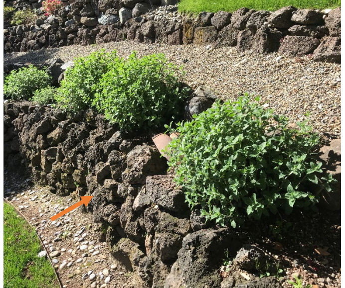
PHOTO 5: Terraced and drained retaining walls
