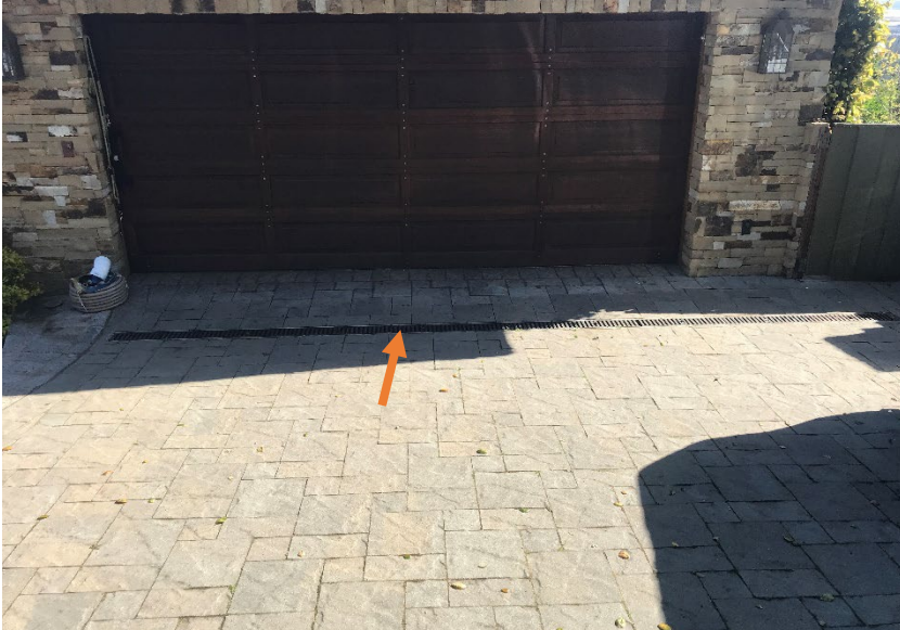
PHOTO 1: Trench drain at end of driveway
