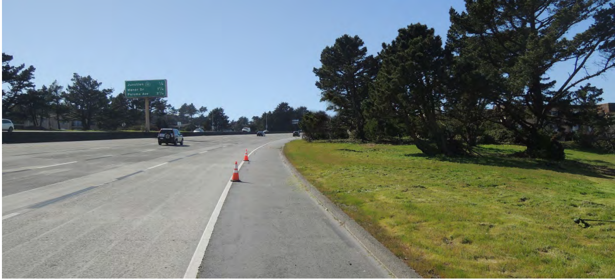
Figure 1-30 Existing Conditions at Location 10
