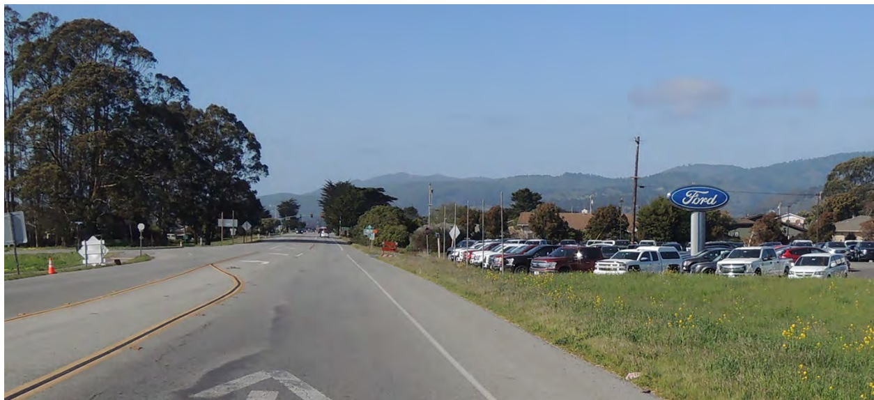
Figure 1-5 Existing Conditions at Location 2
