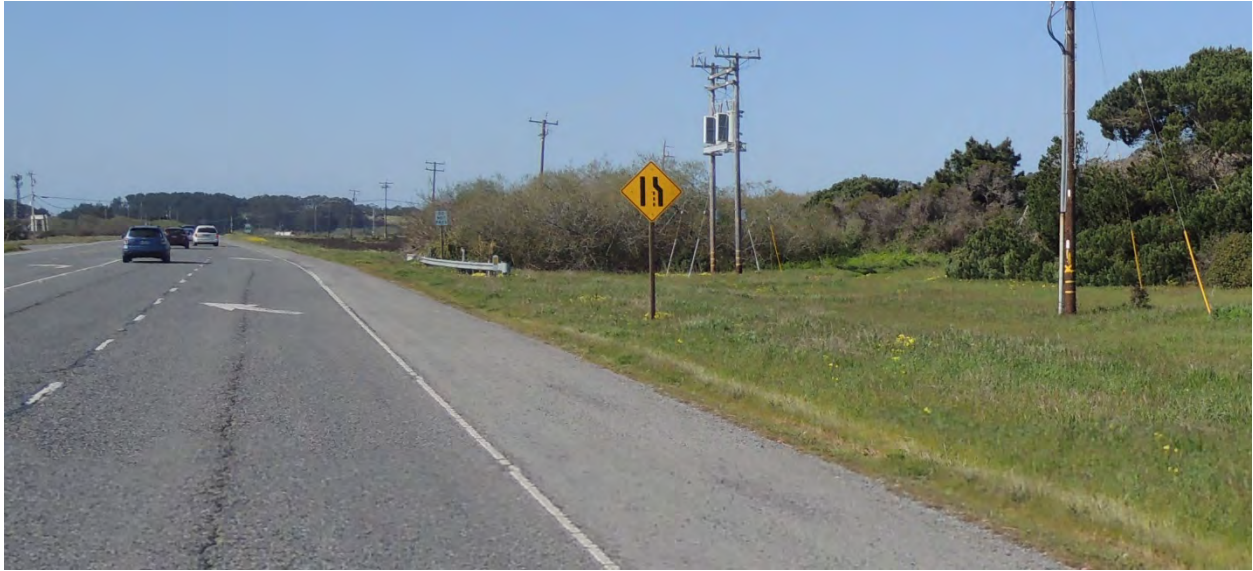
Figure 1-17 Existing Conditions at Location 6
