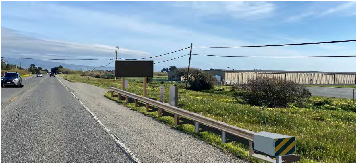
Figure 1-14 Visual Simulation of VMS (shown without message displayed) and MGS at Location 5
